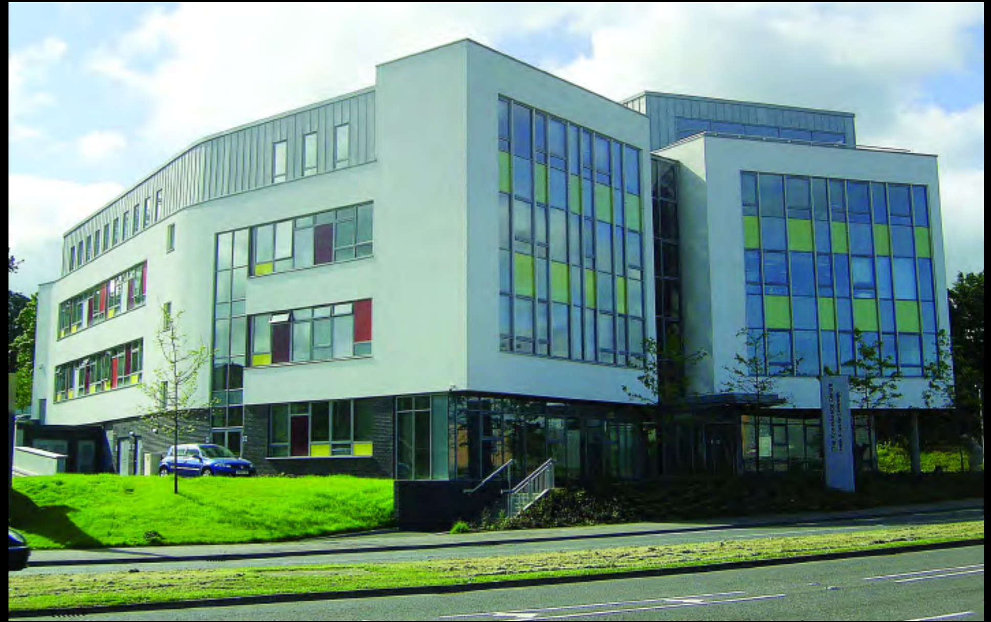
CASE STUDY: Knockbrea Health Centre
