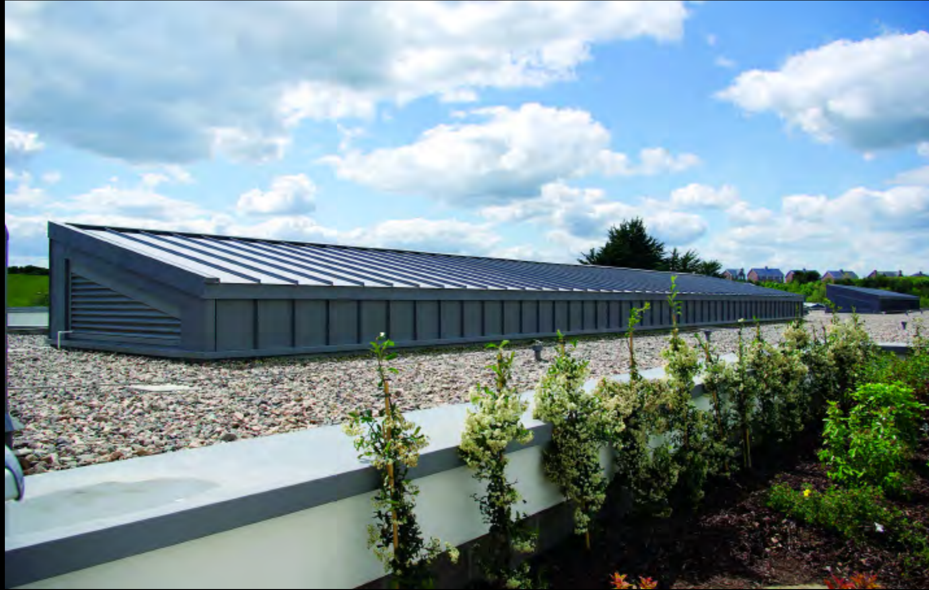
CASE STUDY: Downshire Hospital, Downpatrick
