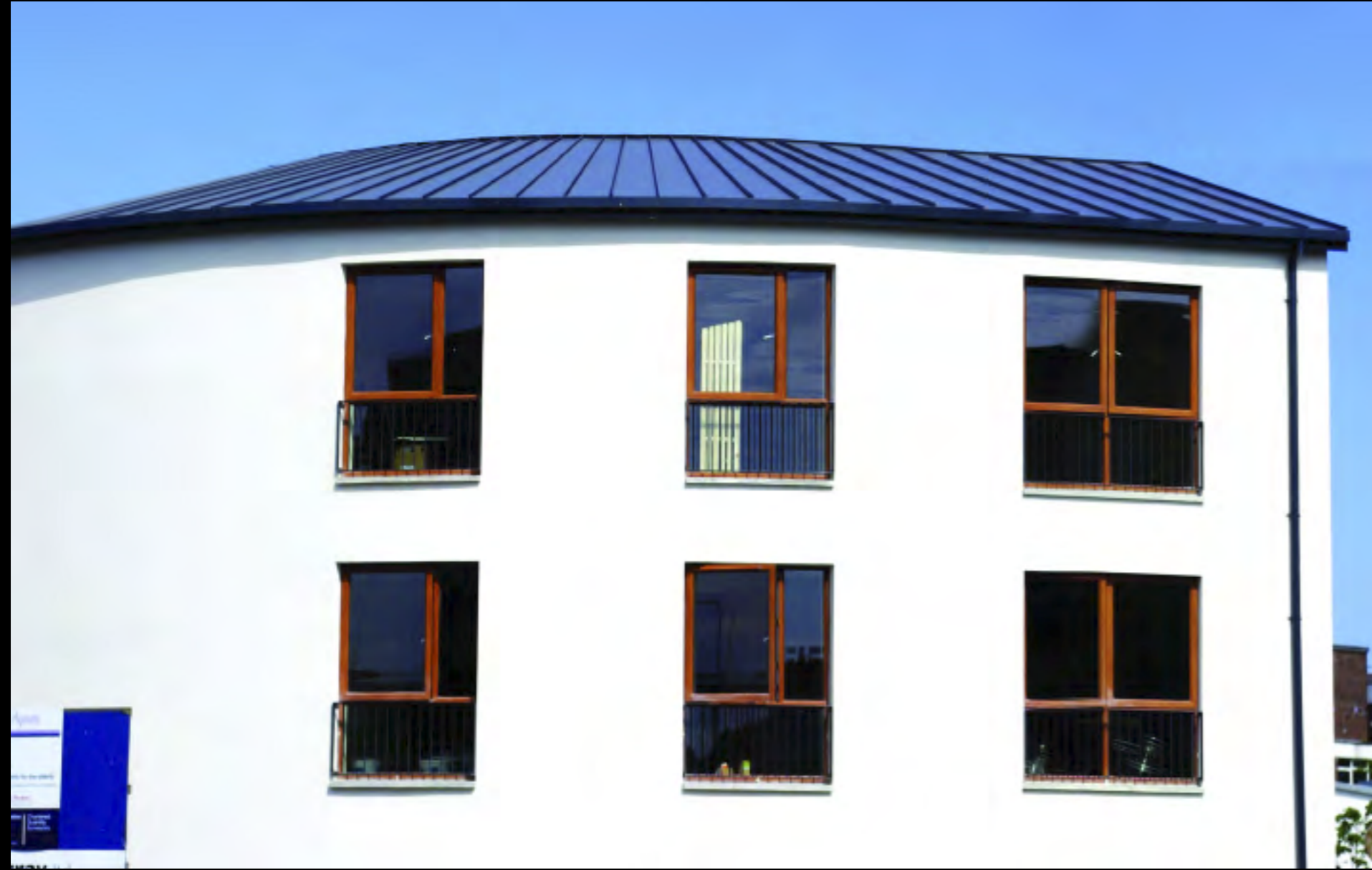
CASE STUDY: Hamilton Road Apartments, Bangor
