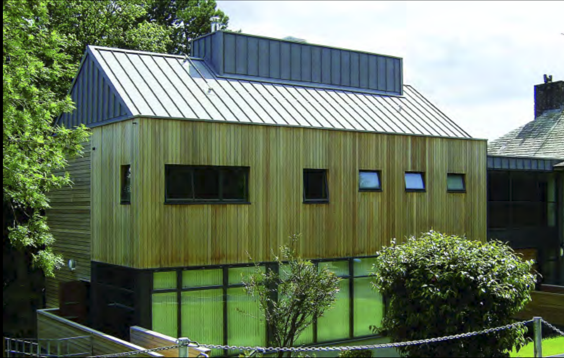
CASE STUDY: Shannagh-more Outward Bound Centre, Newcastle ARCHITECTS: Todd Architects
